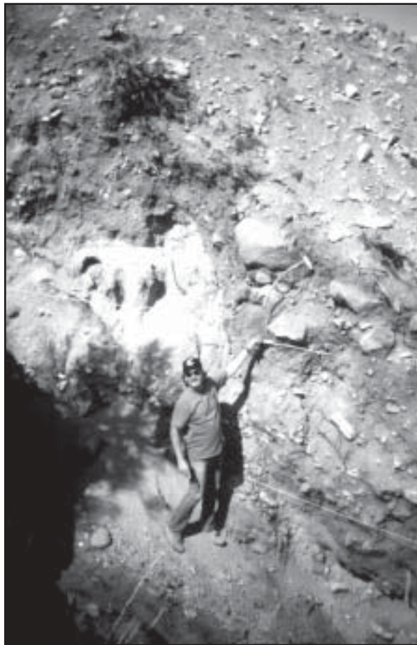
Figure 2. Backhoe trench along the Genoa fault near Walley's Hot Springs, south of the town of Genoa, Douglas County. The maximum displacement along the fault during its last event, about 550 to 650 years ago, was 18 feet (Ramelli and others, 1999). See www.nbmg.unr.edu/dox/sp27.pdf for Nevada Bureau of Mines and Geology Special Publication 27, a booklet on Living with Earthquakes in Nevada, for more information about earthquake hazards.
