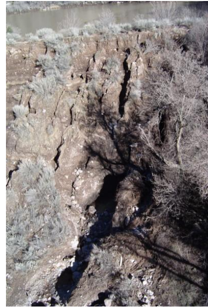
Figure 3-3 Schroeder Dam in Beaver Dam State Park. Erosion cut into the front face of the earthen dam.
